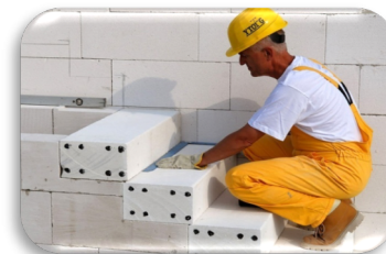
Ytong Block Factory
