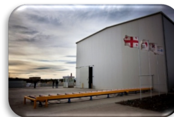
Sandwich Panel Factory
